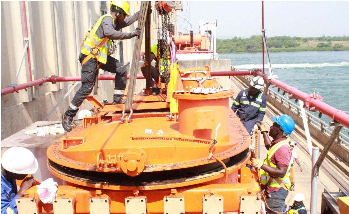
Regasketing of Unit 1 transformer completed successfully
