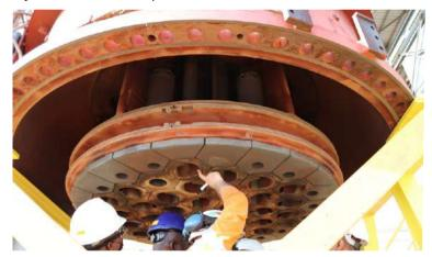
The inspection was also aimed at assessing the rotor condition, carrying out a visual inspection of the compressor, recalibrating, adjusting, replacing or repair of parts and correction of instrument settings as per the agreed work scope. It also involved the implementation of upgrades as per the agreement between VRA and GE, as well as reporting gas turbine generator condition, including recommendations for future operation and maintenance. This is to ensure reliability of power supply to
