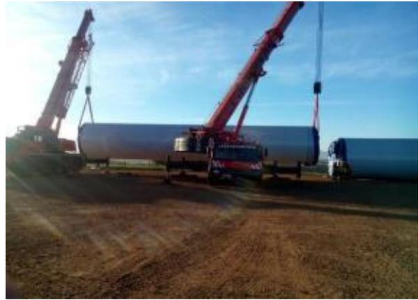
**Figure 3-2: Transportation of a Tower section**
